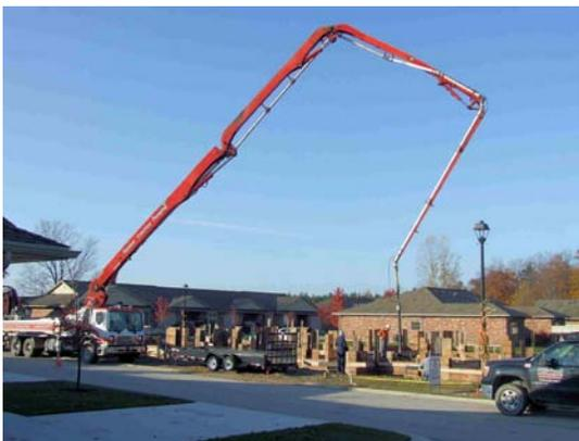
**After the infloor heating tubes are in place, the concrete floor is poured using a pumper truck to precisely direct the concrete.**
