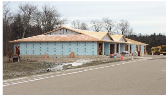
Outside wall insulation
