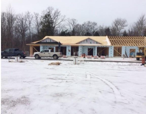
Roofing has started
